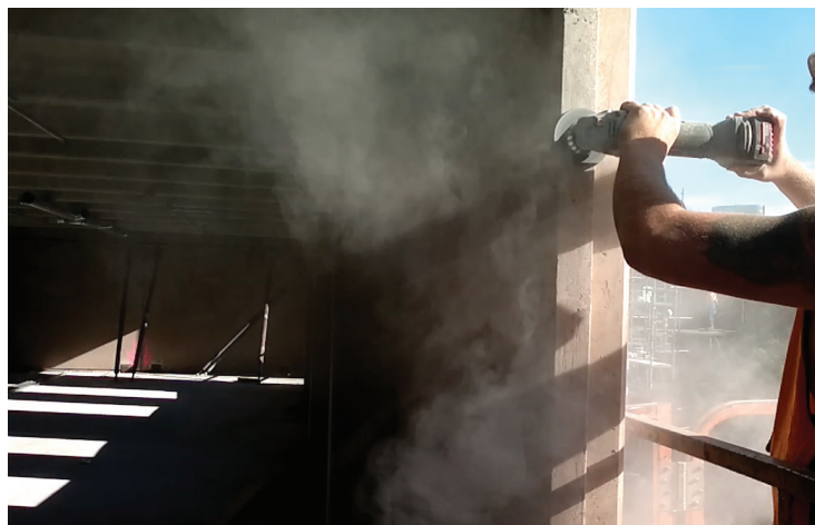
Early stage - preparations for where the façades will be placed
