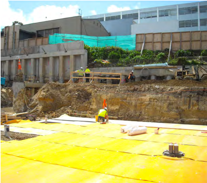
SikaProof® Bentonite - below ground waterproofing membrane. Chosen for its speed of installation, ability to self-heal and excellent peel adhesion to poured concrete – even in damp conditions.
