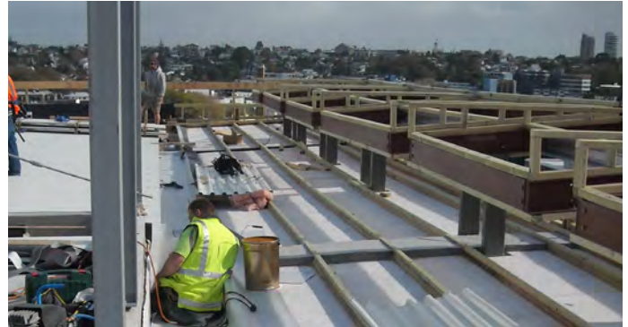
Sarnafil® G410-20L Felt - Chosen for the deck and gutter applications due to its 2mm thickness and ability to detail easily.
